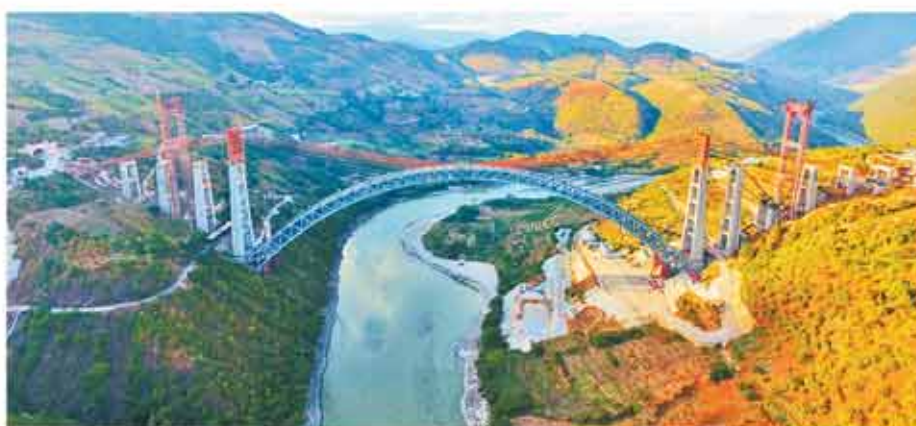
Aerial photo taken on Dec. 9, 2018 shows the railway arch bridge across the Nujiang River in southwest China's Yunnan Province. With a grand arch bridge erected on Monday morning, Chinese constructors have built the longest-spanning railway arch bridge with a single span of 490 meters. The bridge is a key project of the 220-km-long Dali-Ruili railway which is a key section of the China-Myanmar international railway corridor linking Kunming, the provincial capital of Yunnan, with Yangon of Myanmar. Photo by Xinhua
