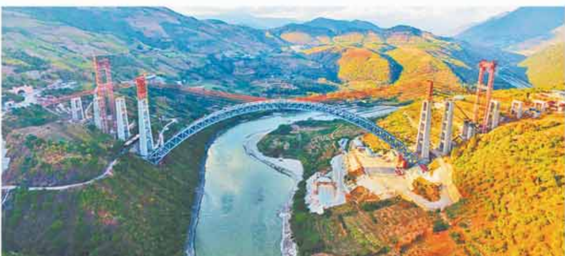
Aerial photo taken on Dec. 9, 2018 shows the railway arch bridge across the Nujiang River in southwest China's Yunnan Province. With a grand arch bridge erected on Monday morning, Chinese constructors have built the longest-spanning railway arch bridge with a single span of 490 meters. The bridge is a key project of the 220-km-long Dali-Ruili railway which is a key section of the China-Myanmar international railway corridor linking Kunming, the provincial capital of Yunnan, with Yangon of Myanmar
