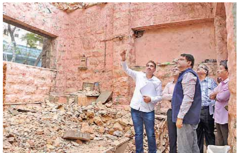
Principal Secretary Arvind Kumar and other officials inspecting the restoration works at Mozamjahi Market on Saturday
