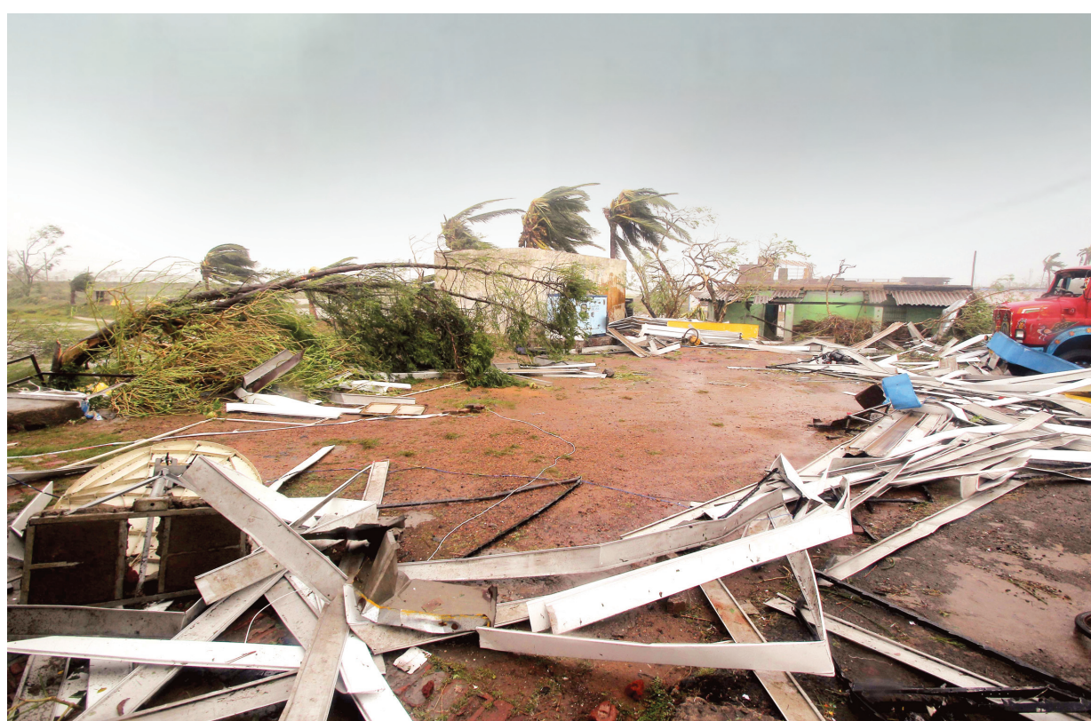
Damaged structures and uprooted trees lie along a road in Puri after Cyclone Fani hit Odisha on Friday
