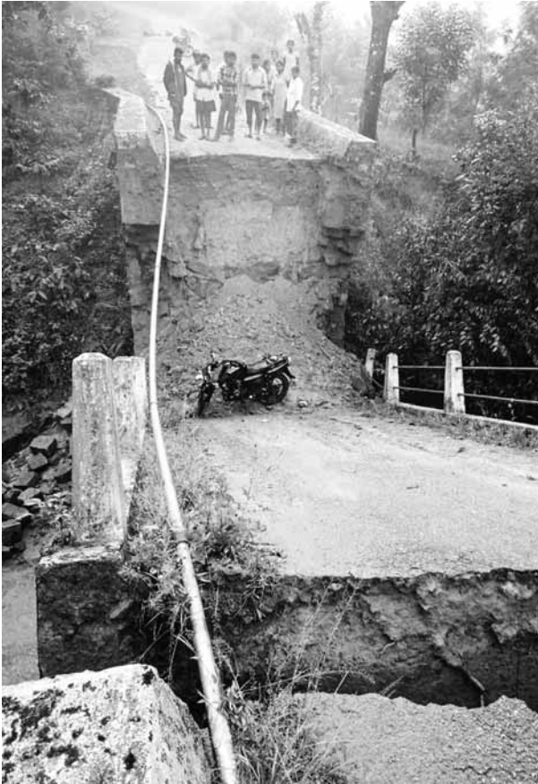
A view of a damaged bridge due to landslide following rain in Chikmagalur PTI
