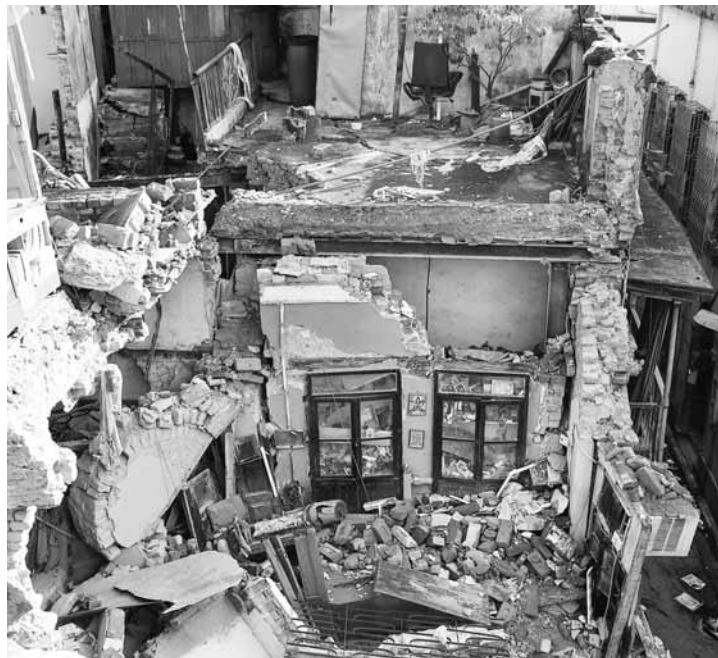
A view of a damaged building in Bowbazar area, where several houses have been damaged owing to tunnel boring for East-West metro corridor in Kolkata on Sunday
