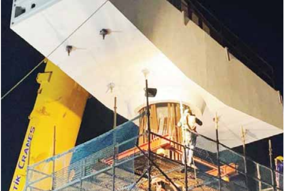
Uttar Pradesh Rail Metro Corporation placing the first 'Cross Arm' at IIT Kanpur station on Wednesday.
