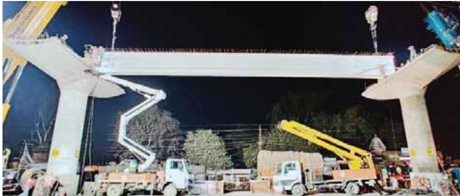
Kanpur Metro places the first "I" Girder at IIT-K metro station.
