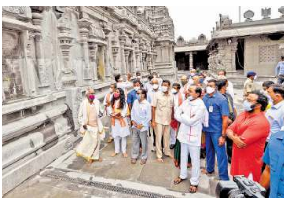
Chief Minister K Chandrashekhar Rao inspecting Yadadri temple structures under construction on Sunday.
