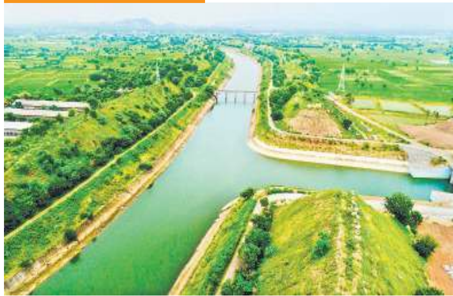
Aerial view of Srisaigam Flood Flow Canal. With the pumping of waters from Kaleshwaram Lift Irrigation Project into the SRSP flood flow canal, there is abundant water all along 160-km flood flow canal
