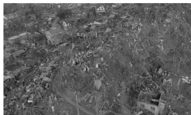
In this photo provided by the Philippine Navy, damaged houses and toppled trees lie in Dinagat Island, Surigao del Norte province, southern Philippines on Friday. AP
