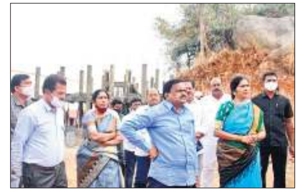
MLA Padma Devender Reddy, Medak District In-charge Collector Venkatrami Reddy and others inspect Mission Bhagiratha works in Ramayampeta municipality on Tuesday
