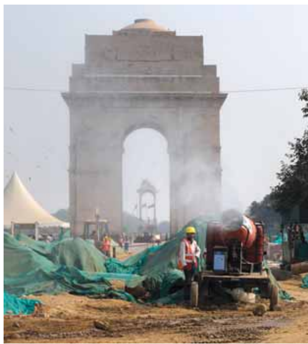
A worker uses an anti-smog gun to control dust at a construction site at the landmark India Gate monument in New Delhi
