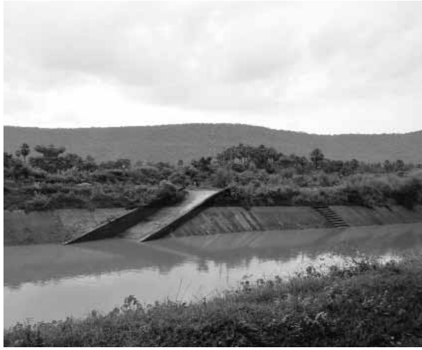
Animal-friendly ramp at Kulei on Rengali Main Canal
