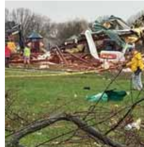
were immediately associated with the collapse.
