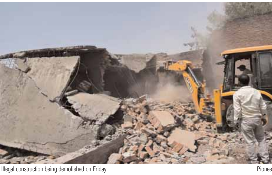
Illegal construction being demolished on Friday. Pioneer.
