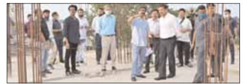
CM Hemant Soren inspecting the under construction building at Jagannathpur, Dhurwa in Ranchi on Monday. PNS
