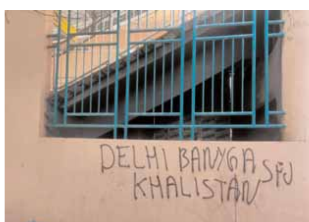
A slogan on the walls of Shivaji Park Delhi Metro station. Ranjan Dimri/Pioneer
