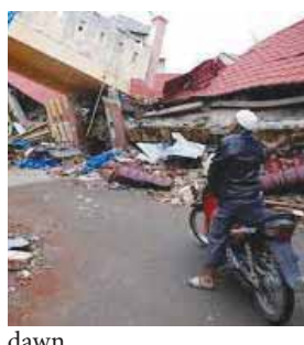
Damage from an earthquake in Bali.
