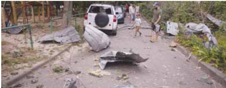
Local residents pass by debris in Kyiv on Wednesday that fell down from their damaged house after a Russian massive rocket attack
