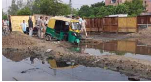
The ditch was dug by the Public Works Department to erect a pillar as part of the construction of a flyover. Monsoon rain which hit the city last week filled the ditch with water. Delhi BJP president Virendra Sachdeva and MP Manoj Tiwari met the family members of auto driver Ajit Sharma, a resident of Nand Nagri, and expressed condolences on behalf of the people of Delhi and the BJP. They also presented a cheque of assistance from the BJP to the family members. On this occasion Naveen Shahdara District BJP President Manoj Tyagi, BJP leader Vikram Mittal and other workers were present. Tiwari said the Arvind Kejriwal government has never paid attention to the development of the North East parliamentary constituency in the last nine years and he would try that the education of the children of late auto driver is not be interrupted and demanded that action should be taken against the officials of the Public Works Department responsible for the accident. In a statement, the AAP government said the Delhi Government has taken cognisance of the incident and is dealing with it very seriously.
