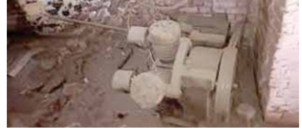
found dead at the spot, he said. Later, one of the injured died at the hospital, the DCP said. The blast had taken place in the air compressor tank used in the plastic moulding machine. The factory was being operated in a rented accommodation of around 150 square yards, Tirkey said. Naresh, the owner of the property, had rented the premises to one Yadav, who was running the factory. Efforts are being made to contact both of them. Their mobile phones
