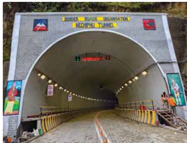
The newly-inaugurated Nepochu Tunnel constructed by Border Roads Organisation in West Kameng district on Tuesday PTI
