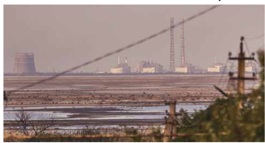
File: The Zaporizhzhia nuclear power plant, Europe's largest, is seen in the background of the shallow Kakhovka Reservoir after the dam collapse, in Enerгодar, Russian-occupied Ukraine, on Tuesday
