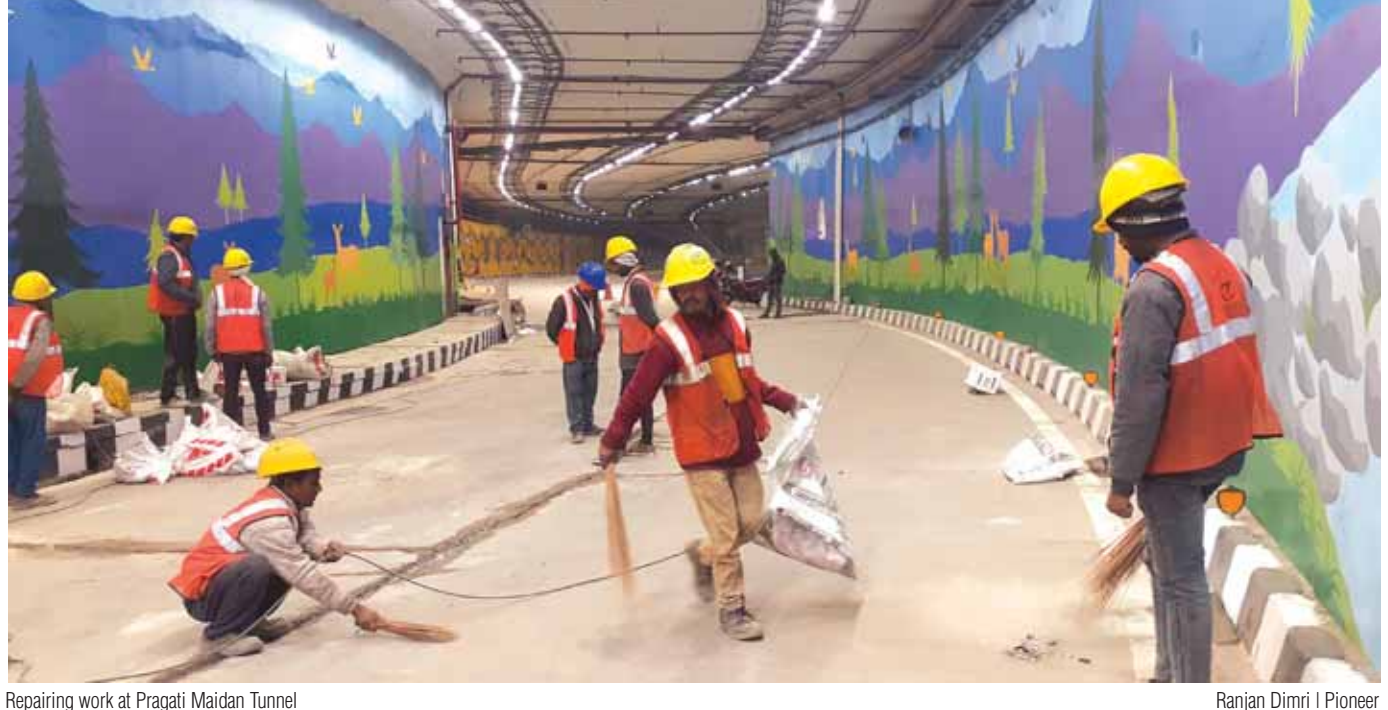
Repairing work at Pragati Maidan Tunnel
