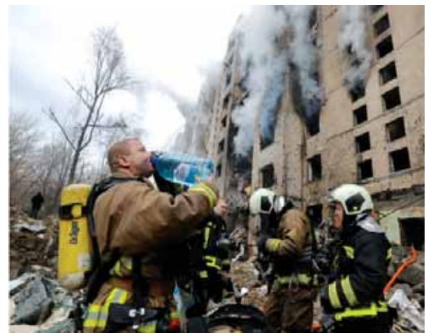
Rescuers work at the site of a damaged building after a missile strike in Kyiv, Ukraine, January 2, 2024.
