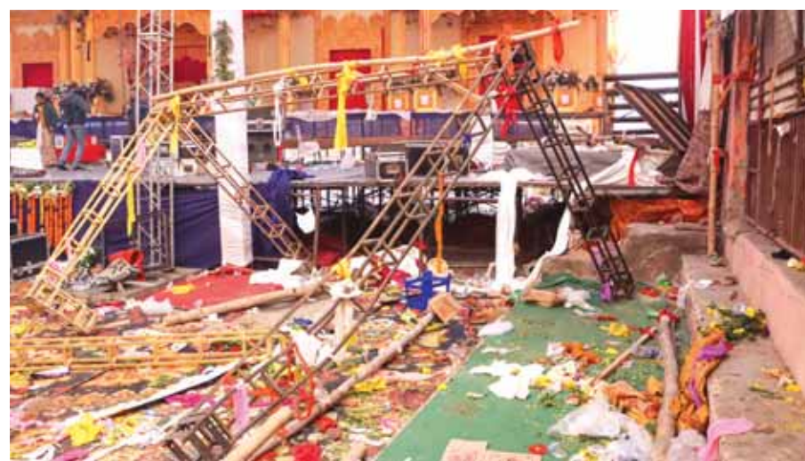
A collapsed platform at Kalkaji Mandir, in New Delhi, on Sunday. At least one person was killed and 17 others suffered injuries after the platform collapsed during a jagran programme, according to officials PTI
