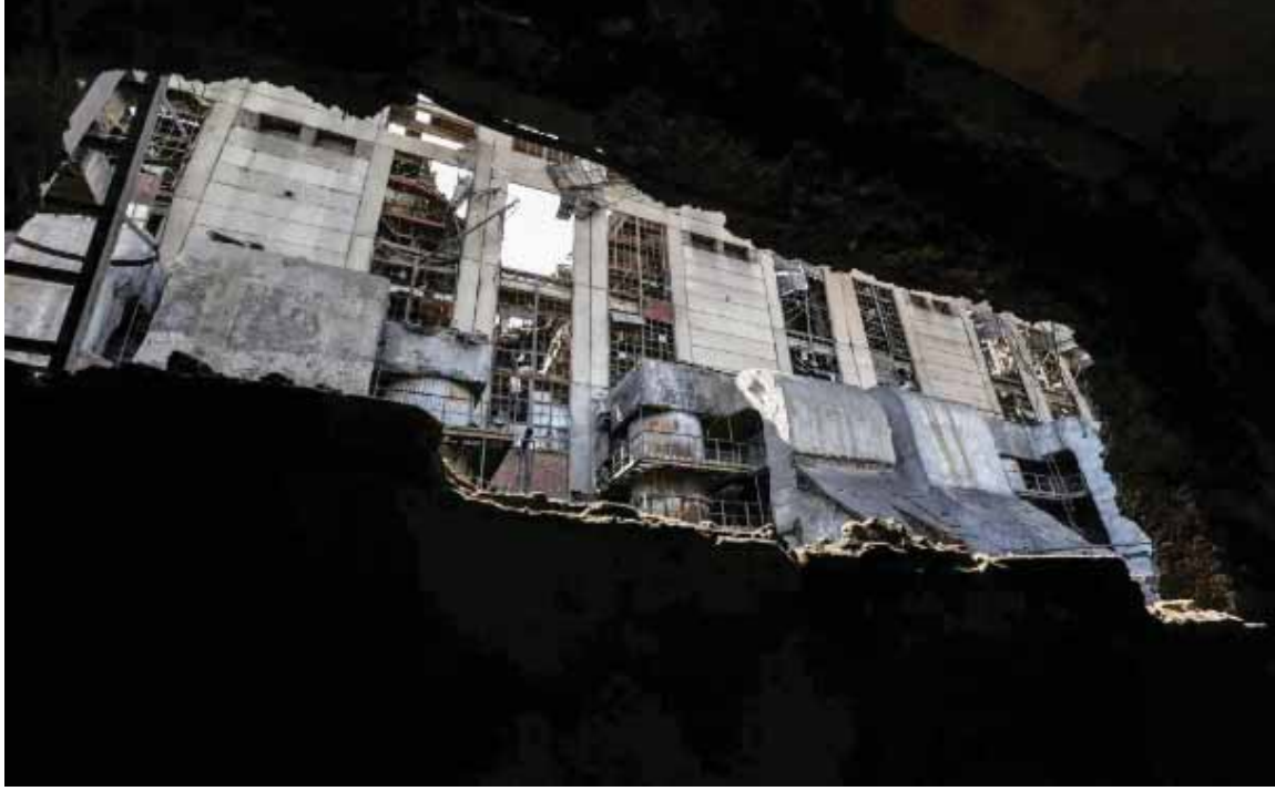
A thermal power plant damaged by a Russian missile strike, amid Moscow's attack on Ukraine, at an undisclosed location in the west of the country in May.
