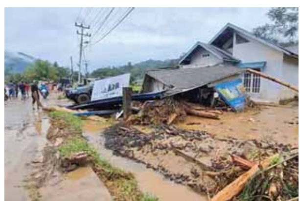
In this image made from video, damaged houses are seen in a village affected by flash flood in Langgai, West Sumatra, Indonesia, Sunday.
