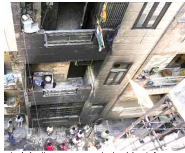
Chief of Delhi Fire Services Atul Garg said a call regarding a blaze at a house near the Bank of India, Krishna Nagar was received at 2.35 am. "The flames were doused by 7.20 am and it was found that the fire began in 11 two-wheelers in the stilt parking of the house and spread to the first floor. The building comprises ground (stilt) plus four floors," he said. Officials said the second,
