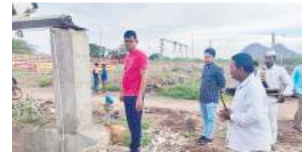
VMC Commissioner Swapnil Dinakar Pundkar inspecting the KL Rao Outfall Drain in Vijayawada on Saturday.
