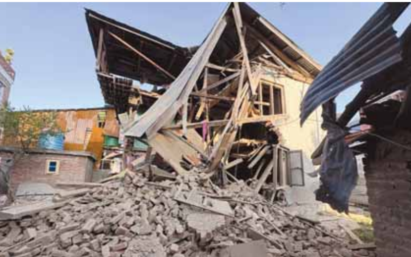
Debris of the house of LeT terrorist Adil Hussain Thokar, which was destroyed after an explosion, in Bithahara, Kashmir PTI
