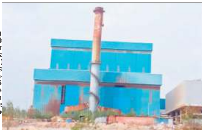
The Waste to Energy plant
