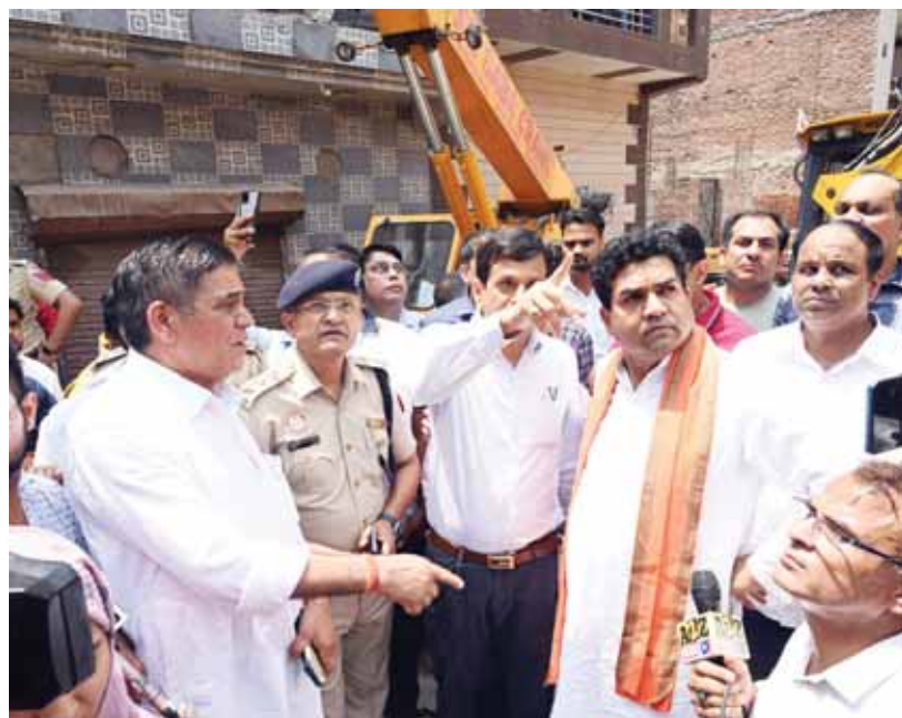
Delhi Minister Kapil Mishra and Dy Speaker in Delhi Assembly Mohan Singh Bisht visit the site of building to take stock of the rescue and relief work in Mustafabad area in New Delhi, ranjan dimri
