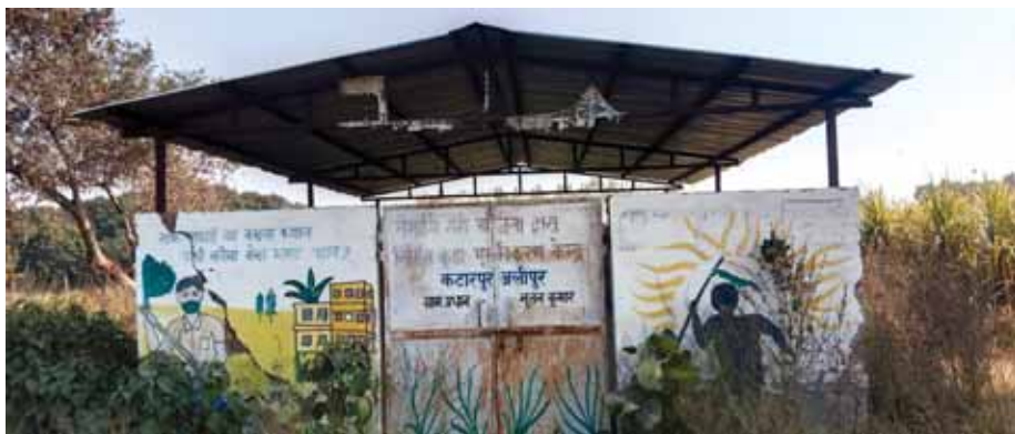
An abandoned garbage collection center in a village along the Ganga
