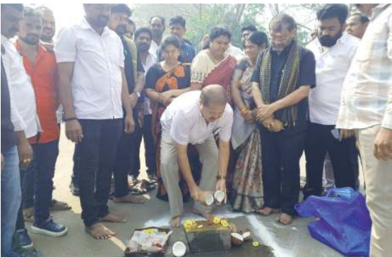
MLA Pantham Nanaji performing bhoomi puja for laying cement concrete road in Kakinada on Thursday
