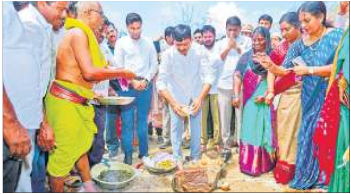
Minister Ponguleti Srinivas Reddy laying the foundation stone for Indiramma houses at Penuballi in Khammam district on Thursday. District Collector Muzammil Khan is also present
