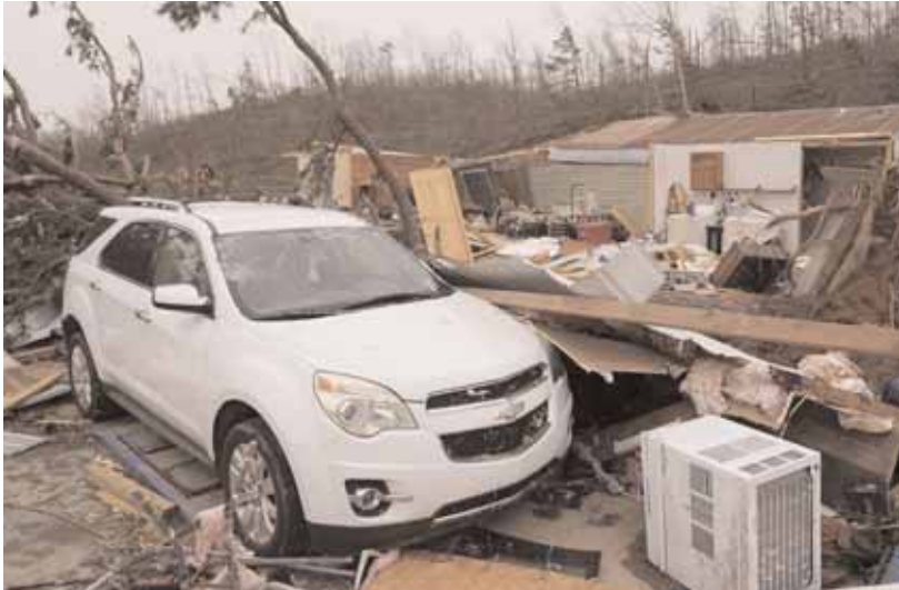
A vehicle sits in front of a damaged home and debris from a severe storm on Saturday in Wayne County. API/PTI
