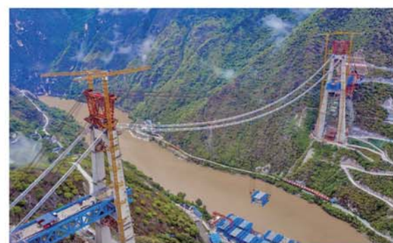
The Jinsha River Bridge on the Lijiang-Shangri-la railway under construction. (Xinhua)
